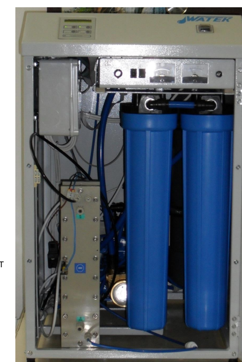
Fully automated IWA 60 EDI system available from WATEK s.r.o. in combination with EDI-Z2-AF module available from MemBrain s.r.o.
